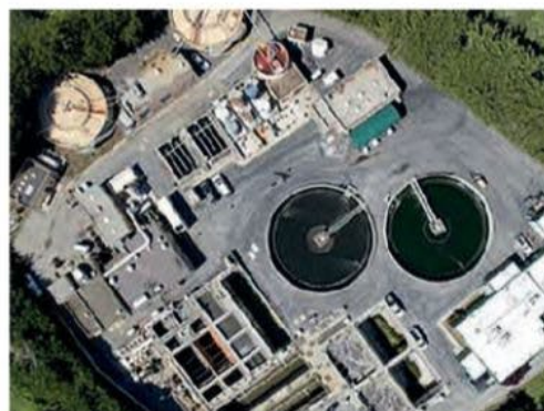
The Sewer Authority Mid-Coastside (SAM) treatment plant where they're using SENTRY wastewater sensors for real-time, early-on influent insight to better manage variable influent from industrial dischargers
