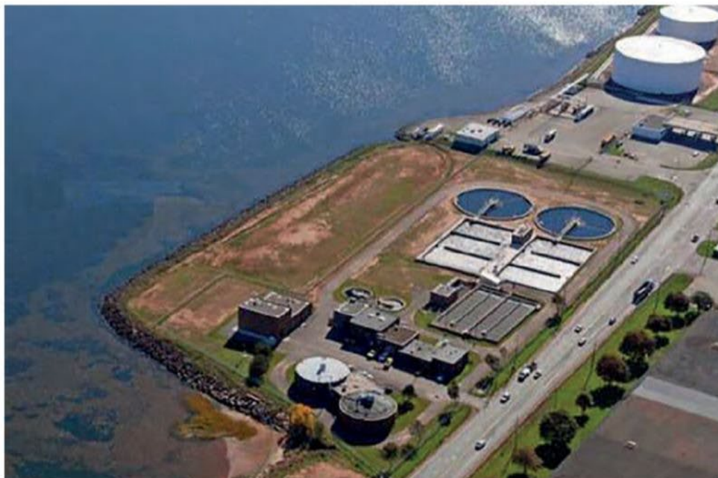
Charlottetown Treatment Plant where they're using SENTRY wastewater sensors upstream to monitor incoming loading and make more accurate aeration adjustments for energy conservation
